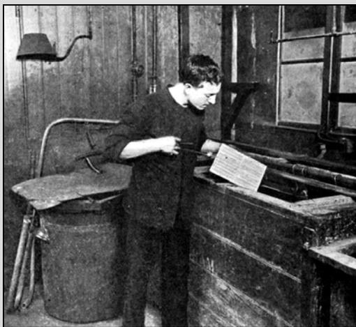
A copper-faced plate about to receive a nickel deposit at printer Eyre and Spottiswoode. Aside from it being a plate instead of a cylinder, little has changed in more than 100 years. The modern-day baths at Saueressig would be instantly recognisable to the young man in this 1913 photo.
