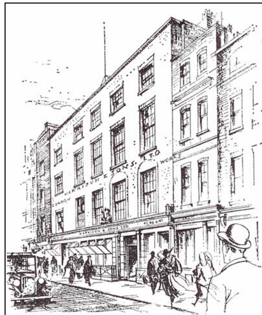
The original St Martin's Lane premises
